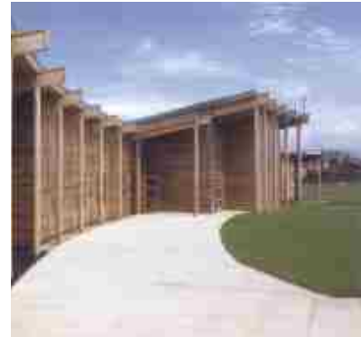
Typical image of new school buildings
